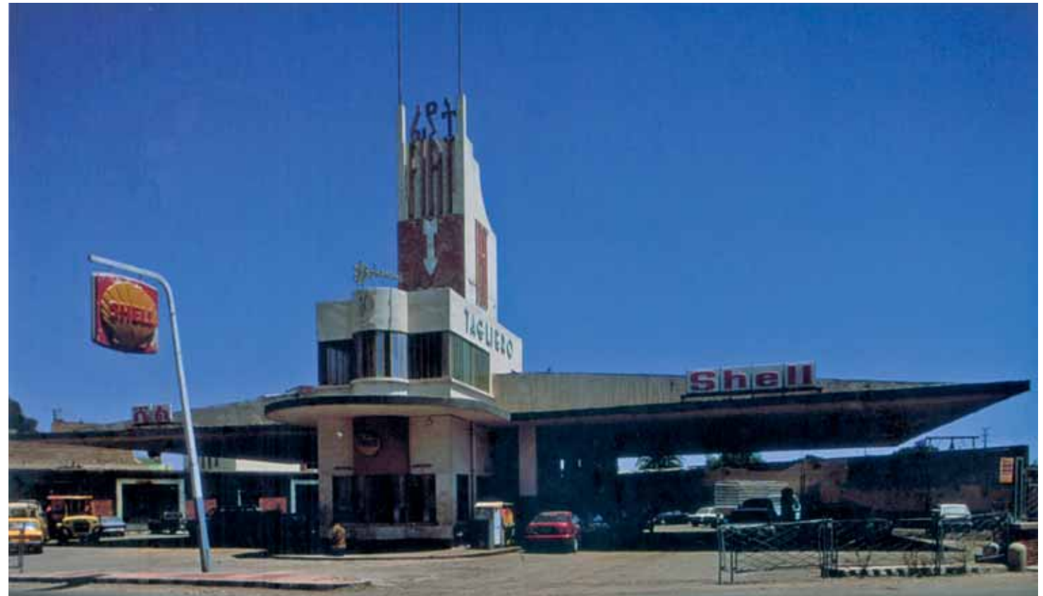
Fiat Tagliero Service station, Engineer Giuseppe Pettazzi, 1938, Photographer Edward Denison
